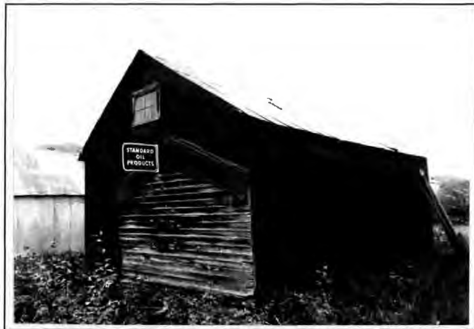
Figure 42. The Donnelley/Standard Oil Warehouse, 1993. The view is looking northeast.
